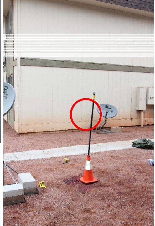
Circled area shows the corresponding impact hole into exterior wall of Building Q, Apartment 161. Forensic analysis identified this recovered bullet to have the same rifling characteristics as test-fired bullets Decedent's Glock .40 caliber handgun
