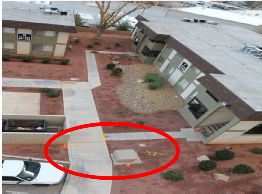
Circled area depicts location of electrical power box where Officer Marsec took cover and dumpster area where Officer Giese took cover at time of shooting
