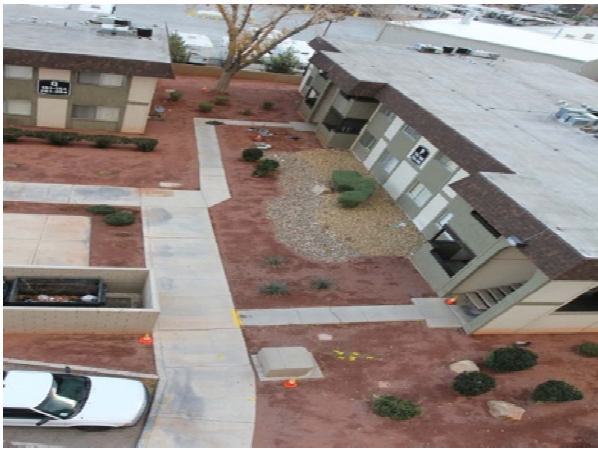
Overview, Building Q (top left) and Building P (right)
